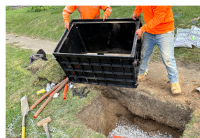
Lift the HandHole and position in place
