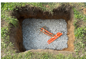
Dig trench, fill bottom w/ recommended drainage.
