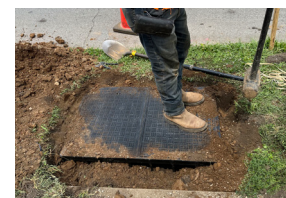
Pack in backfill. Tier 22 Rated
