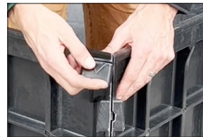
Outside corners: slide on FastClips - 2 per corner*
