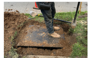
Pack in backfill. Tier 22 Rated
