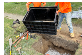
Lift the HandHole and position in place
